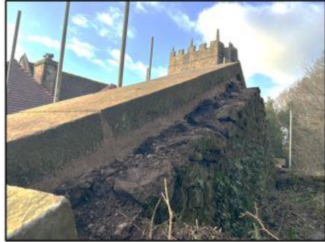
Inner view where the slate roof existed.
